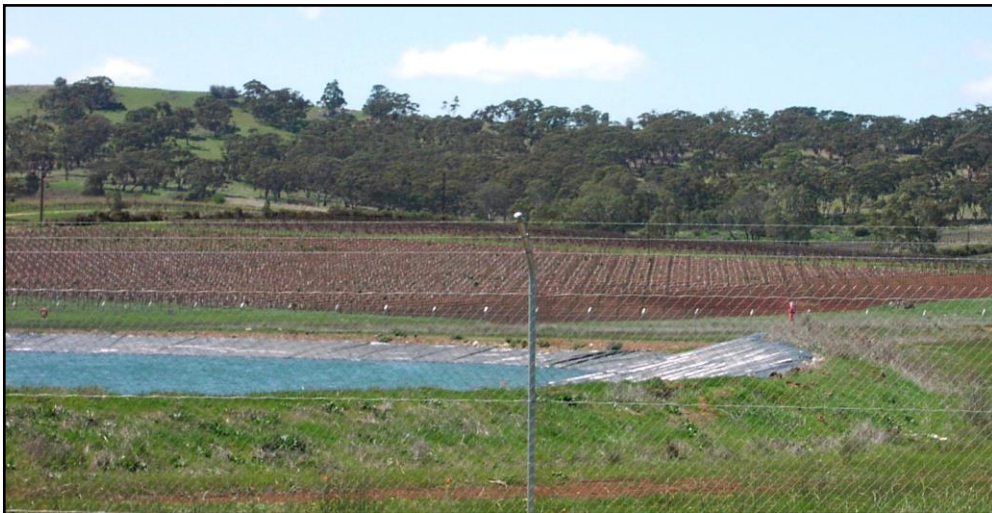
Plaque 4: Another Clare valley irrigation water storage with a very flat internal slope. Note that on this one there is almost zero width at the top of the embankment.
