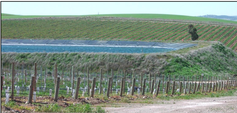
Plaque 2: The same storage as above about a year later. Internal slopes are about 1 on 4. A low slope such as this makes it easy to compact the surface and to roll-out and weld the liner. It also reduces the tendency of the liner to creep down the slope.
