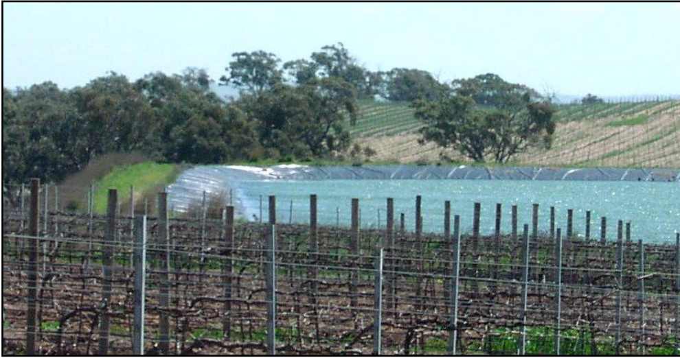
Plaque 3: Another lined irrigation water storage in the Clare Valley. The internal slope on this one appears to be even flatter – about 1 on 5. There is no tension on these liners, so the top edge is simply turned down into a shallow trench and backfilled. Current SA Water standard practice requires that the top of the liner be fixed to a perimetric concrete ring beam all around the storage.
