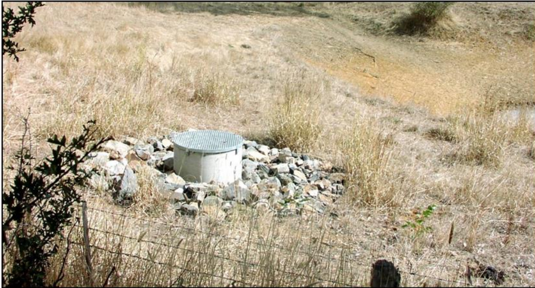
Figure 3 - Typical Small Tank Overflow and Scour Dissipator
