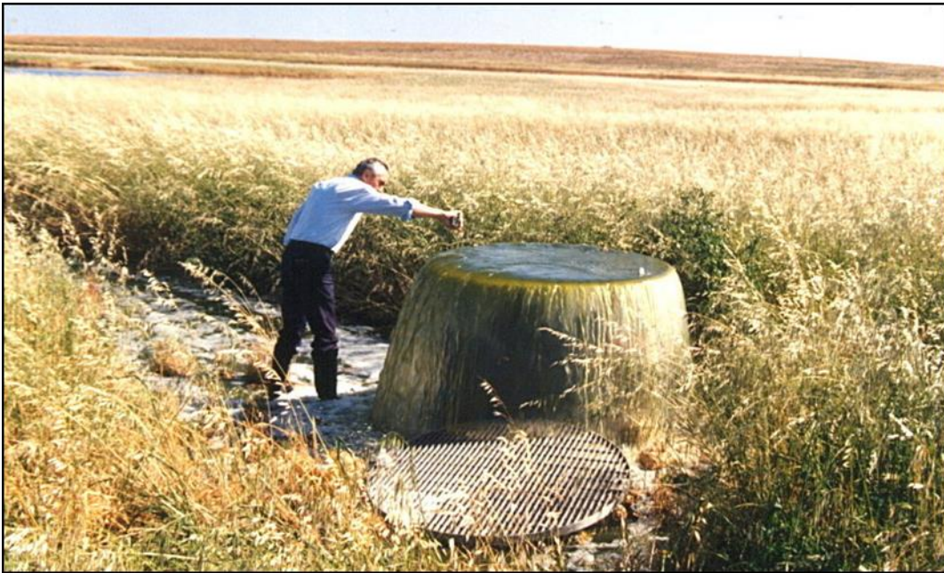
Figure 2 – Murray Bridge WWTP Wetlands Dissipator
